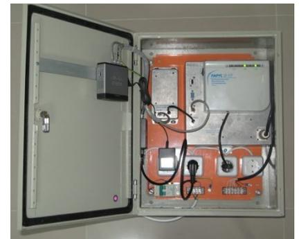
Fig. 6. Field unit of the NSSM system for land installation
