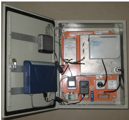
Fig. 7. Field unit of the NSSM system for underground installation
