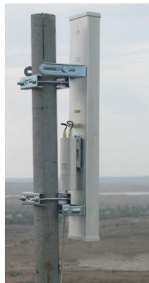
Fig. 10. Access point of the center of a wireless communication network of NSSM
