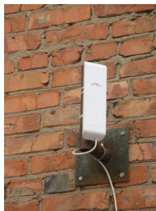
Fig. 11. The client station of a communication network of NSSM for average distances
