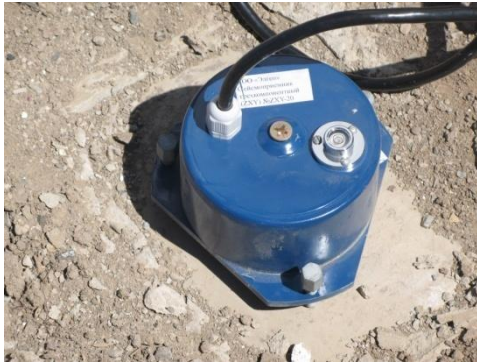
Fig. 6. Installation of the geophone on the concrete foundation
